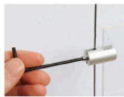
**8** Remove the side screws in the grip connectors, position the wire inside the grooves, and reinstall the side screws.
